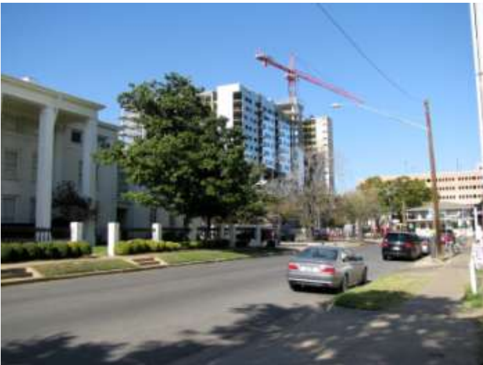
Folks who don't live in Austin any more will be astonished at the new construction going on around the church.
