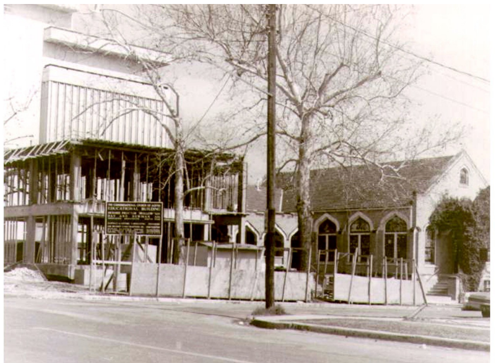
1969 The church in the snow with the education wing under construction
