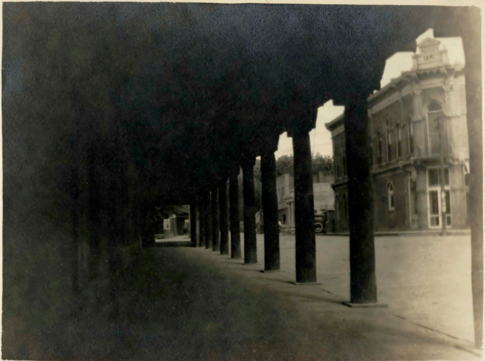
INSIDE THE FACADE OF THE OLD GOVERNORS PALACE SANTA FE
